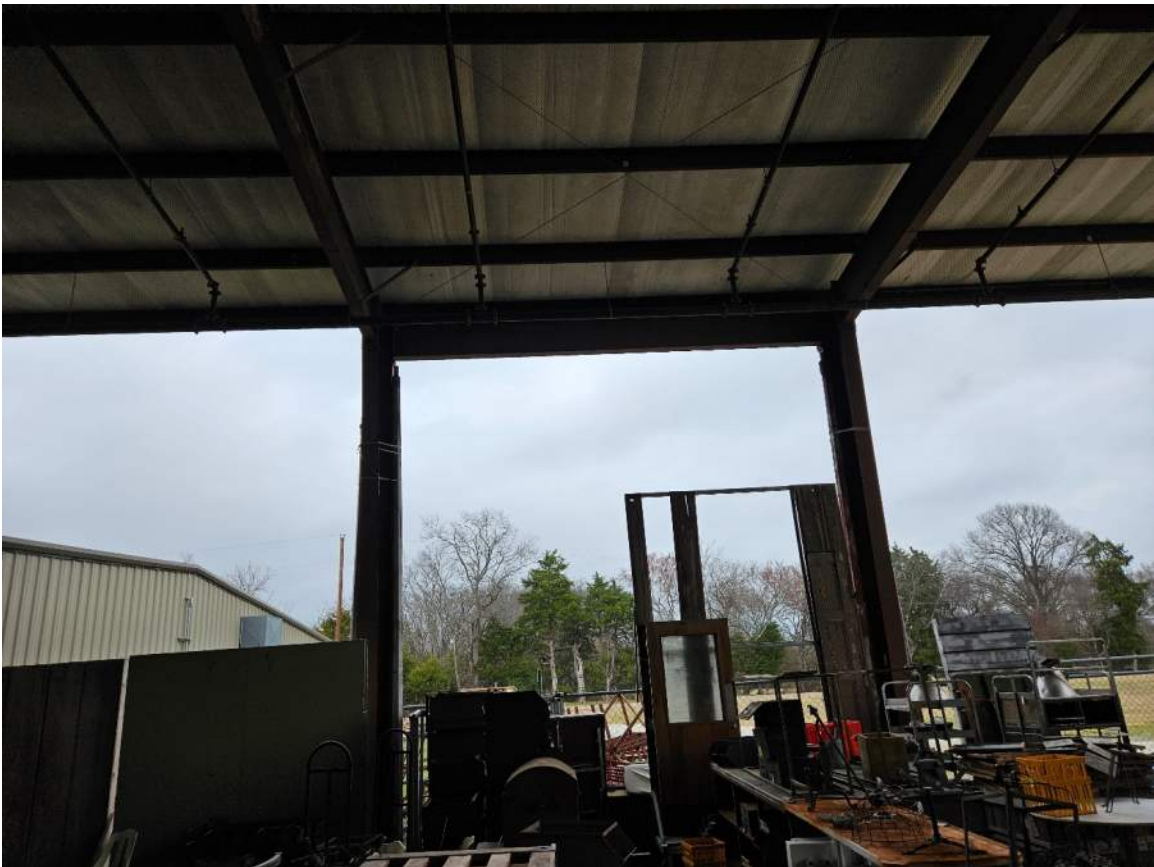
Photo #16 (Portal Frame & Roof "X" Bracing @ Covered Concrete Area – Building 1)
