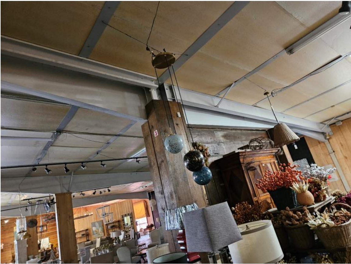
Photo #23 (Indication of add-on or separate build – Building 2)
