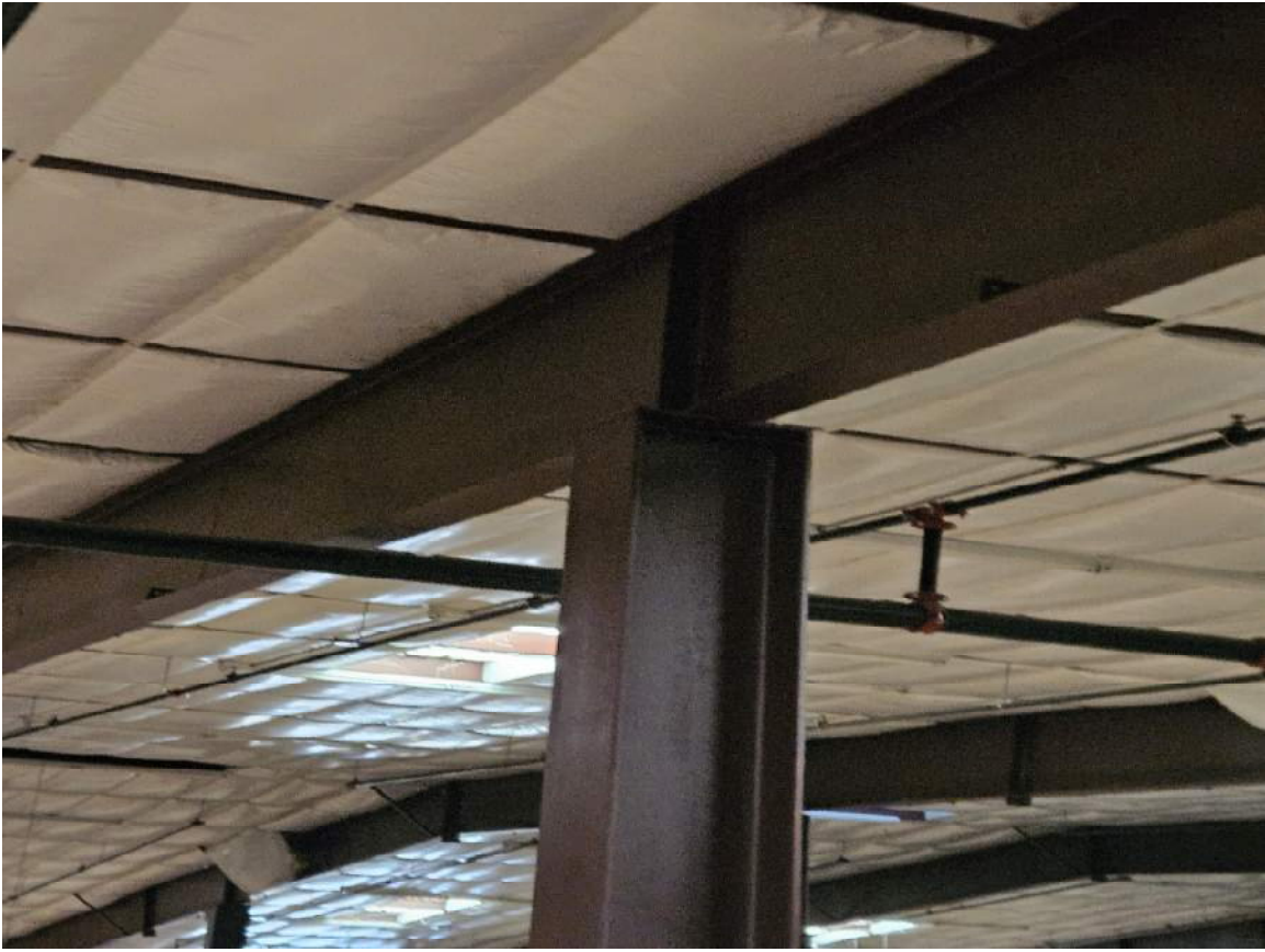
Photo #7 (Typical Interior Column to Rafter Connection – Building 1)
