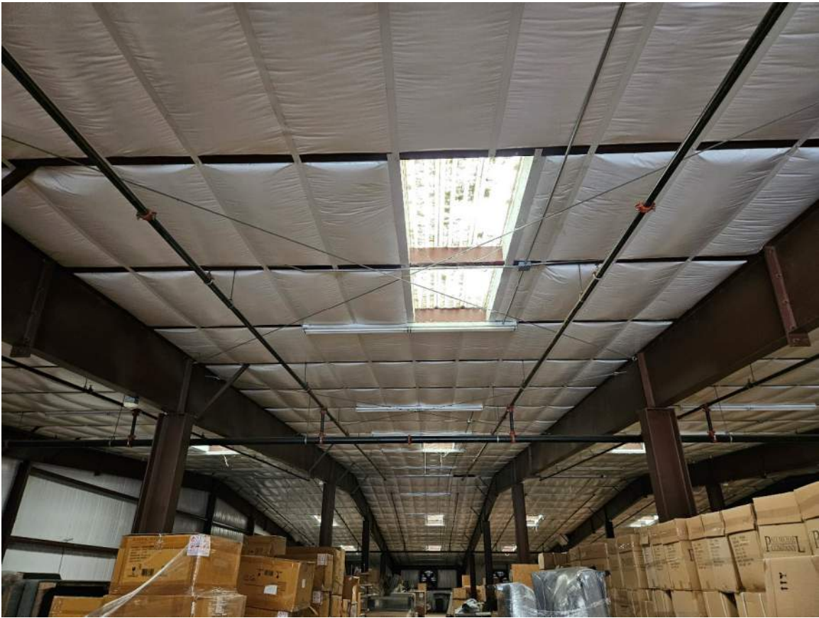
Photo #1 (Roof "X" Bracing – Building 1)
