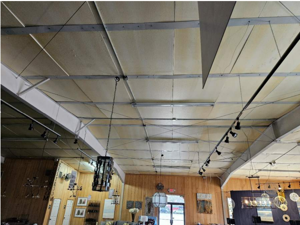
Photo #20 (Roof "X" bracing in one portion – Building 2)
