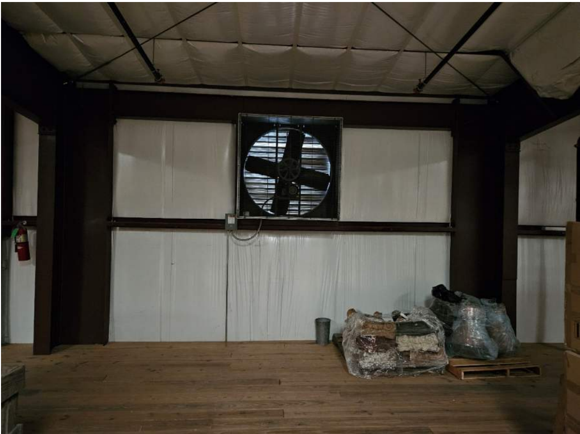
Photo #4 (Portal Frame – Building 1)
