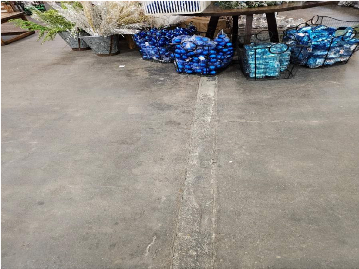
Photo #25 (Indication of add-on or separate build – Building 2)
