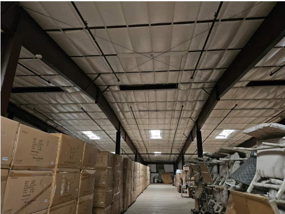
Photo #2 (Roof "X" Bracing – Building 1)
