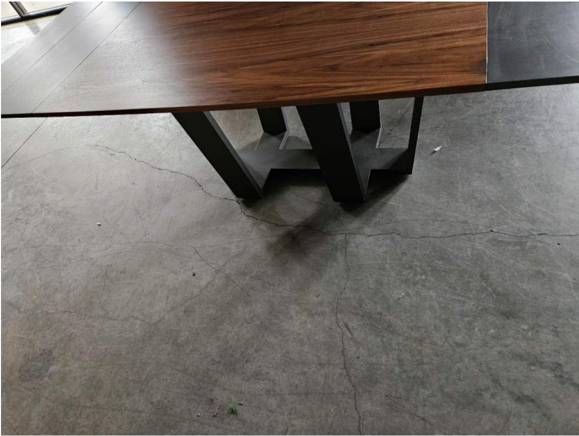
Photo #15 (Concrete Slab Cracking – Building 1)
