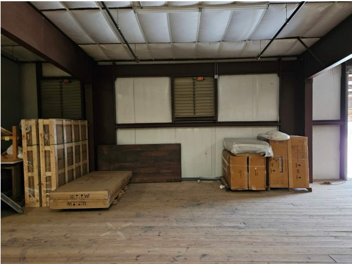
Photo #6 (Portal Frame – Building 1)
