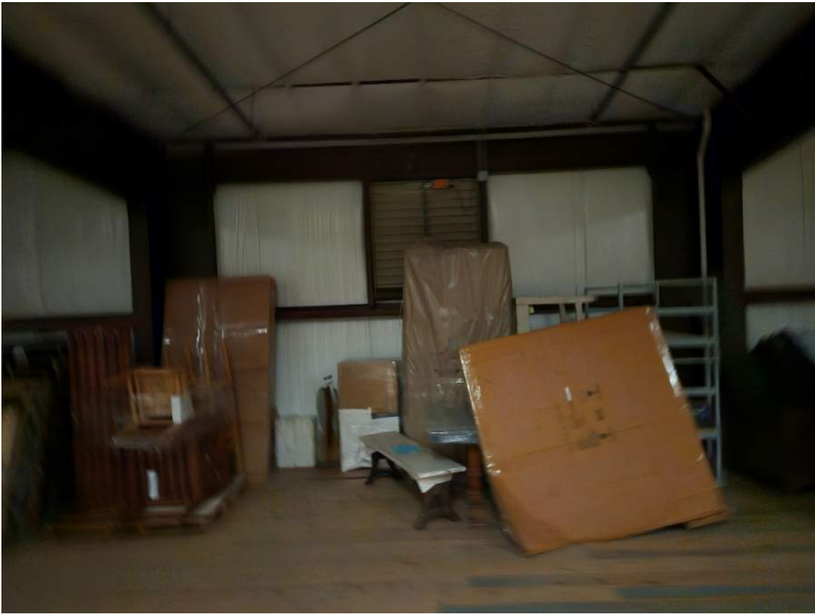
Photo #5 (Portal Frame – Building 1)
