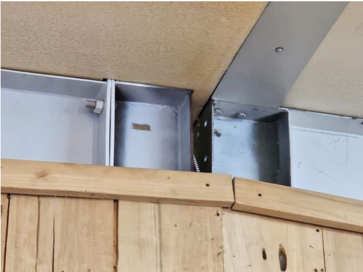
Photo #26 (Indication of add-on or separate build – Building 2)
