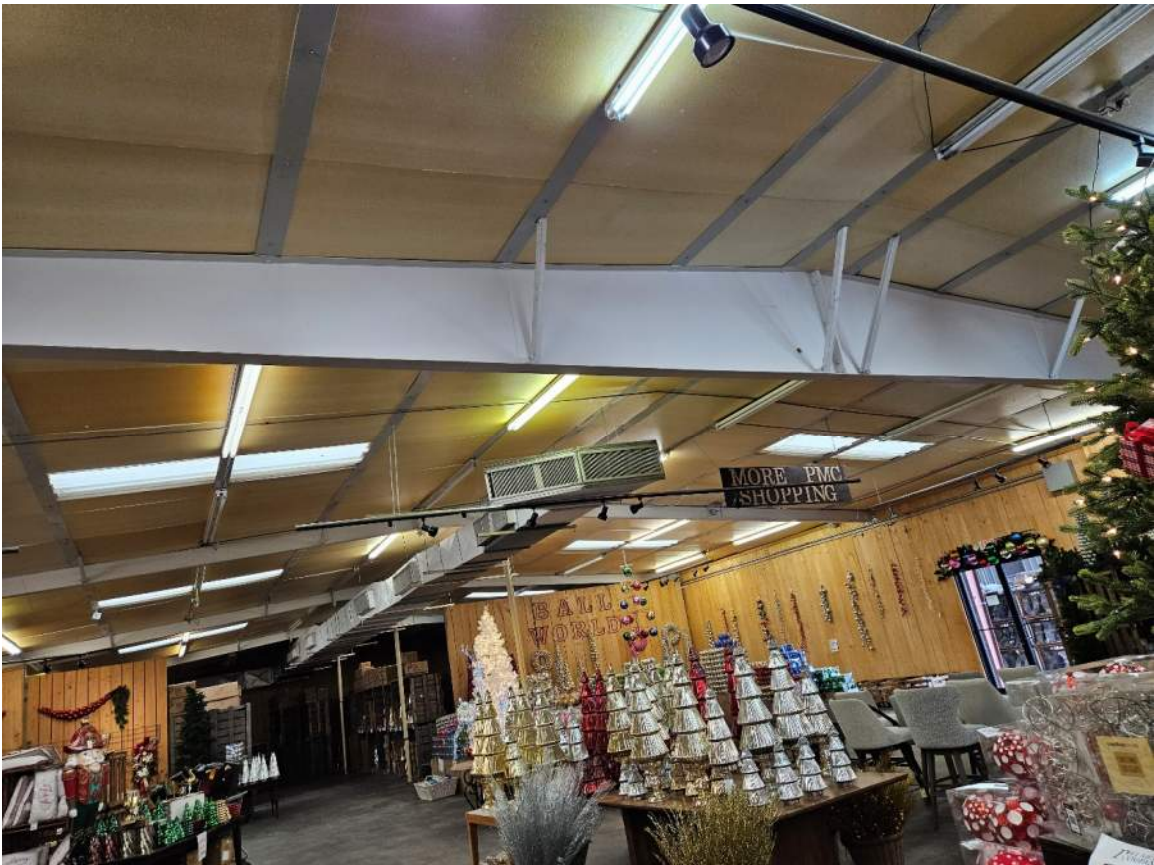
Photo #24 (Indication of add-on or separate build – Building 2)
