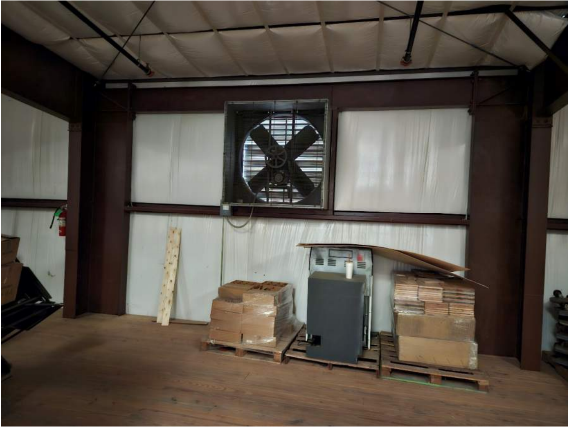
Photo #3 (Portal Frame – Building 1)
