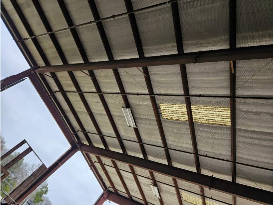
Photo #17 (Portal Frame & Roof "X" Bracing @ Covered Concrete Area – Building 1)
