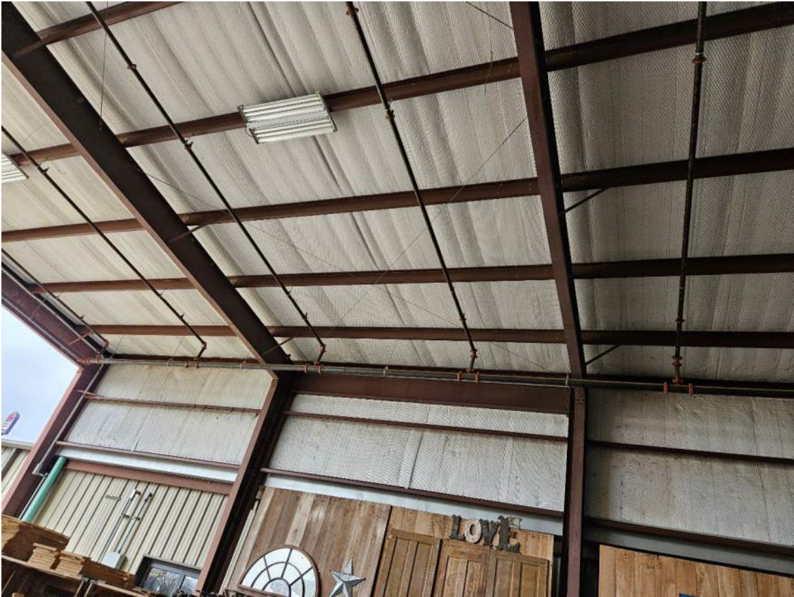
Photo #18 (Portal Frame & Roof "X" Bracing @ Covered Concrete Area – Building 1)
